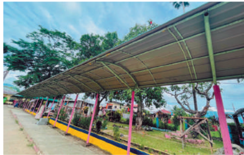
Installation of 100-meter canopy at Sison Elementary School
