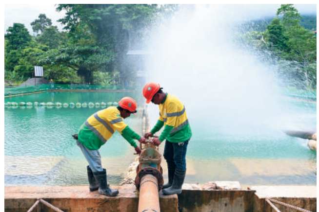
Advance Mine Dewatering activity in the Silangan Project
