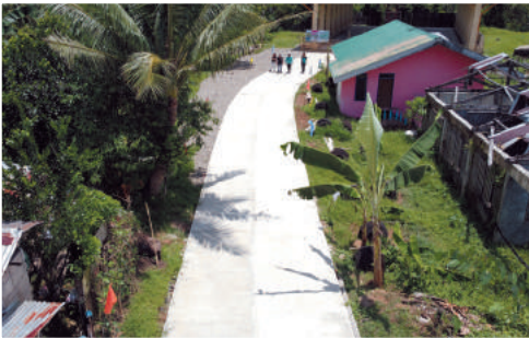
Pathway concreting in Brgy. Upper Patag, Sison
