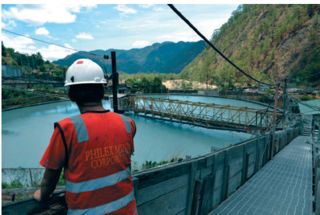
Tailings thickener #2, Padcal Mine's milling process
